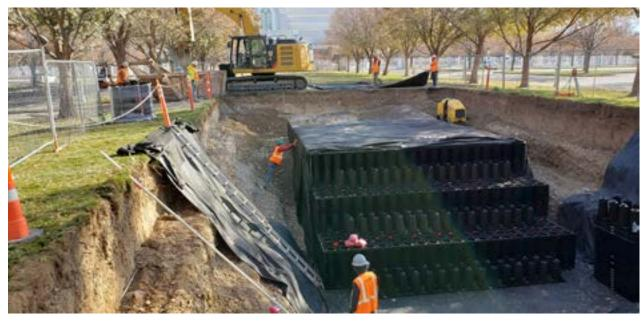
The structural integrity of ACO StormBrixx® allowed for a deeper, 3-layer tank design to meet the capacity and footprint constraints of the project.
