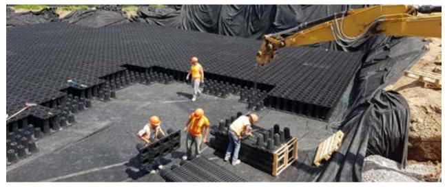
The modular nature of StormBrixx® allowed for an irregular shaped tank to fit the tight site constraints, provide maximum volume, and quick install.
