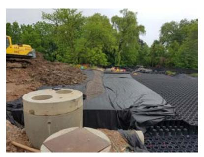
Due to the irregular shape of the tank, twelve (12) StormBrixx® inspection ports were installed to provide access to all corners of the tank for inspections and maintenance
